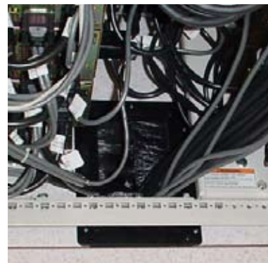
Photo 1. Integral KoldLok Grommet is installed in the raised floor tile providing NFPA required raw metal edge dressing, access to install and remove cables, and sealing around cables to prevent the escape of cooling air
